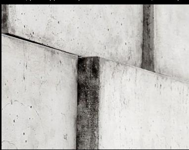
Its weight is 2 kg for 1 cm thick, 5 kg for 2,5 cm and 8 kg for the 4 cm thick, with sort variation between the pieces.
